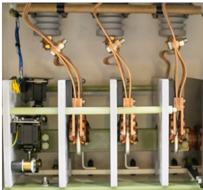
Switch-box with cover removed (primary switch is exposed)
