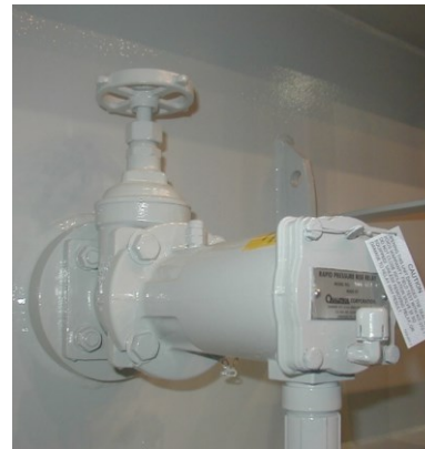
Qualitrol Oil Flange mounted
