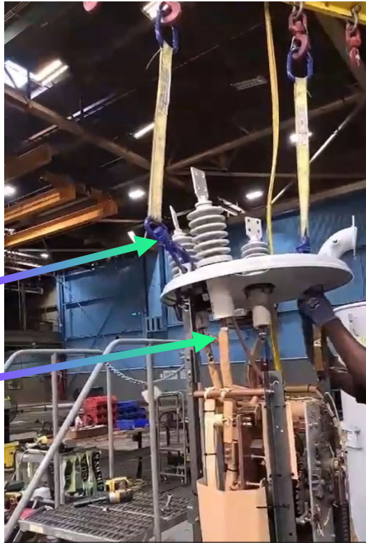
Crane & Lifting Lugs
